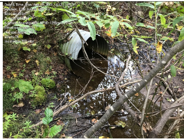
Photo 2. View of the culvert inlet.
