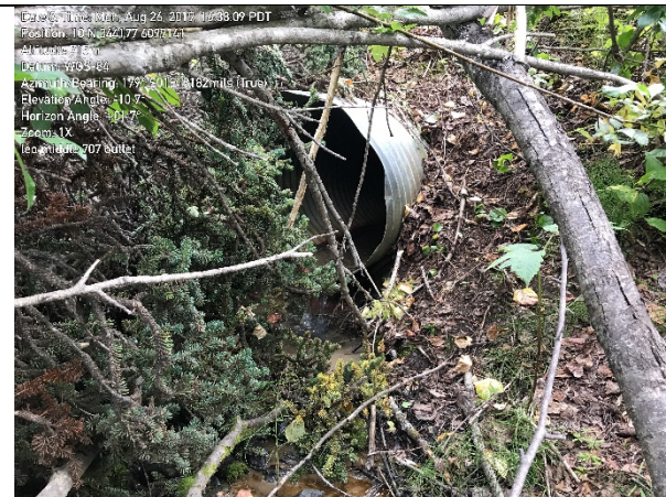
Photo 1. View of culvert outlet with the outlet drop.
